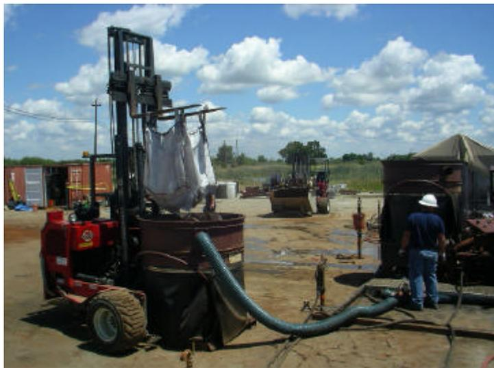
3<sup>rd</sup> Generation Mixing/Blending Unit with Vacuum Dust Control System
