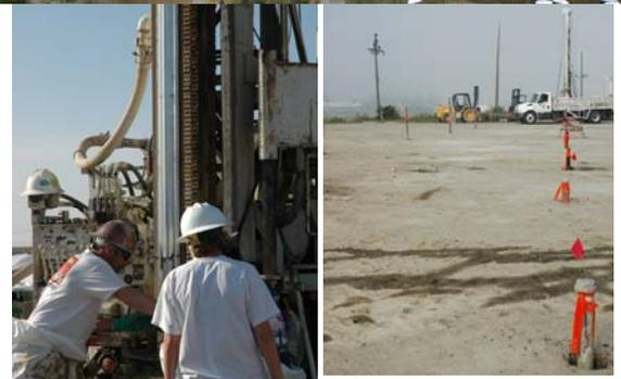
Aerial view of site, installation of frac casings and PRB alignment ready for injection
