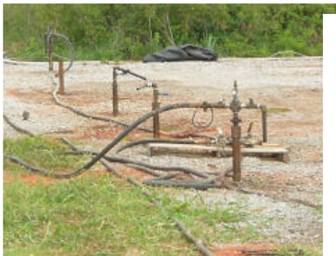
*PRB frac casings along PRB alignment at Tinker AFB, Oklahoma City, Oklahoma*
