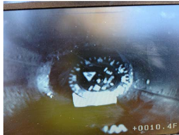
ALIGNING CASING WITH DOWNHOLE CAMERA/COMPASS DURING CASING INSTALLATION
